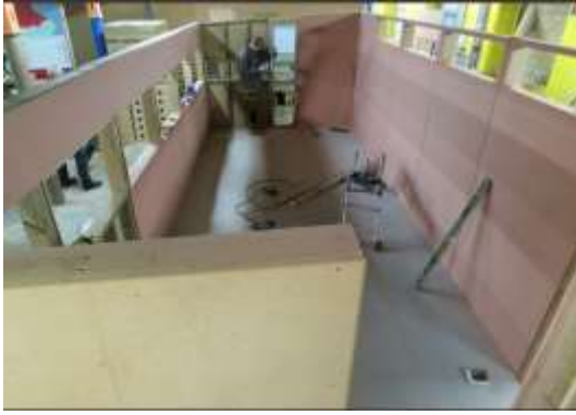
The new hide under construction
